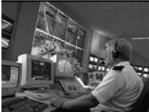
Regional Control Center
