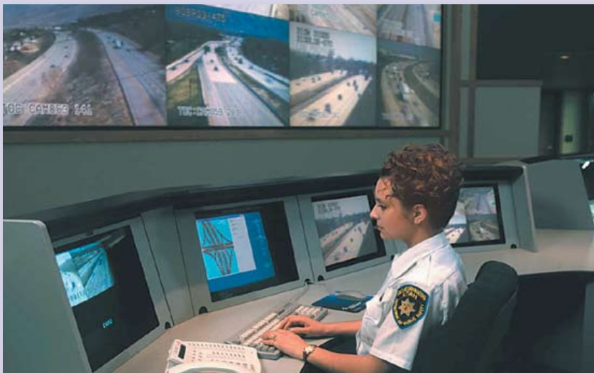
Utah Department of Public Safety Officer accessing the advanced traffic management system, which is integrated with law enforcement’s CAD system.
